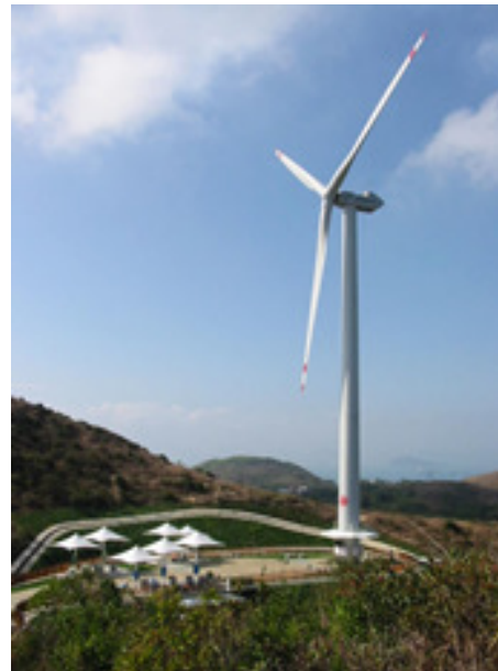
Wind power station
